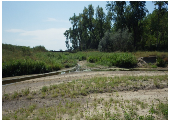
Benson and Patterson Drains. Post augmentation looking south.
