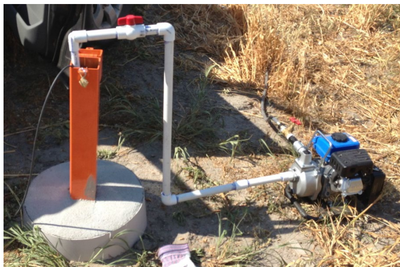
Figure 7. PVC inlet pipe, one-inch clear water pump, and outlet hose
