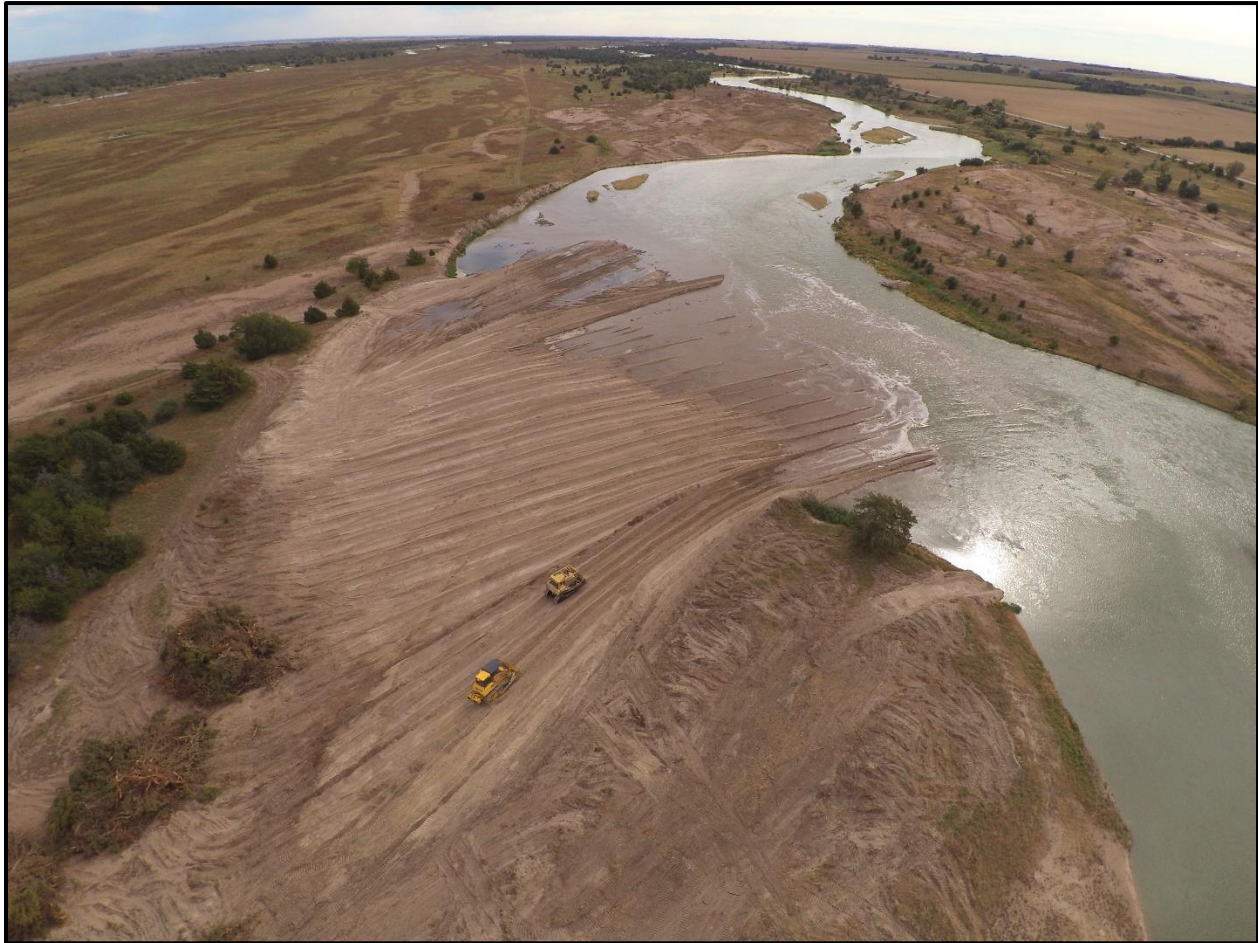
Figure 1.6 Construction of 2019 Sediment Augmentation Project (42,300 yd 3 ).
