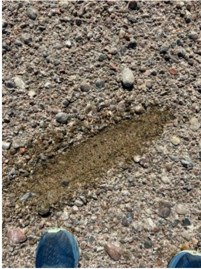
Figure D.4. Visual comparison of coarse armor layer overlaying finer sand on the channel bed approximately 500 feet downstream from the J2 Return
