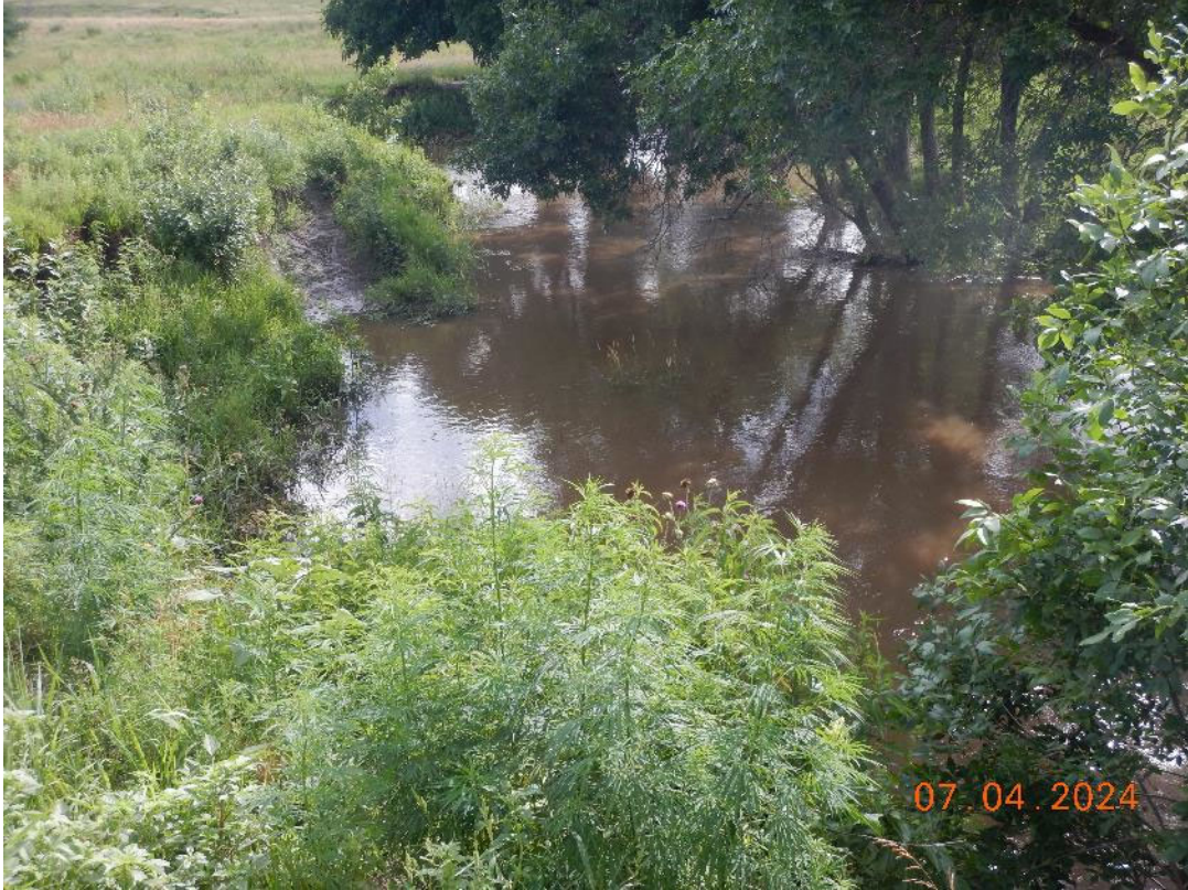
Photograph 13. Looking downstream from County Road 430 culvert.
