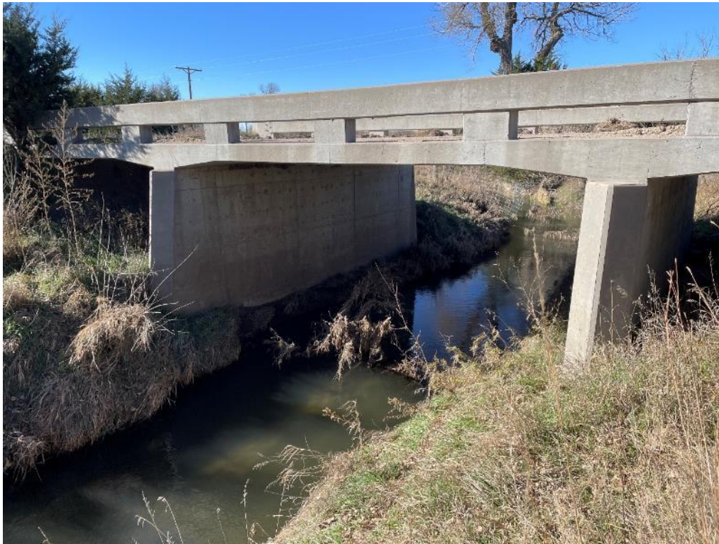
Figure 10: Typical bridge crossing of Plum Creek. Picture from Country Road 435 Crossing.
