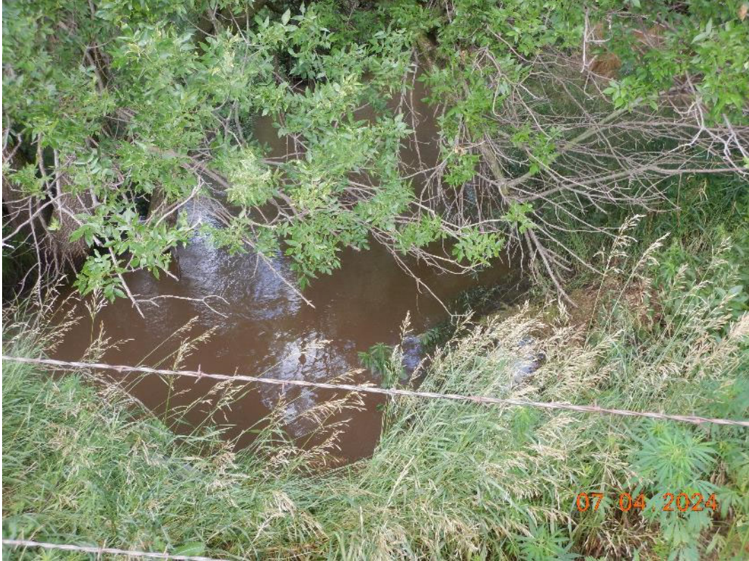
Photograph 11. Looking upstream from County Road 430 culvert.
