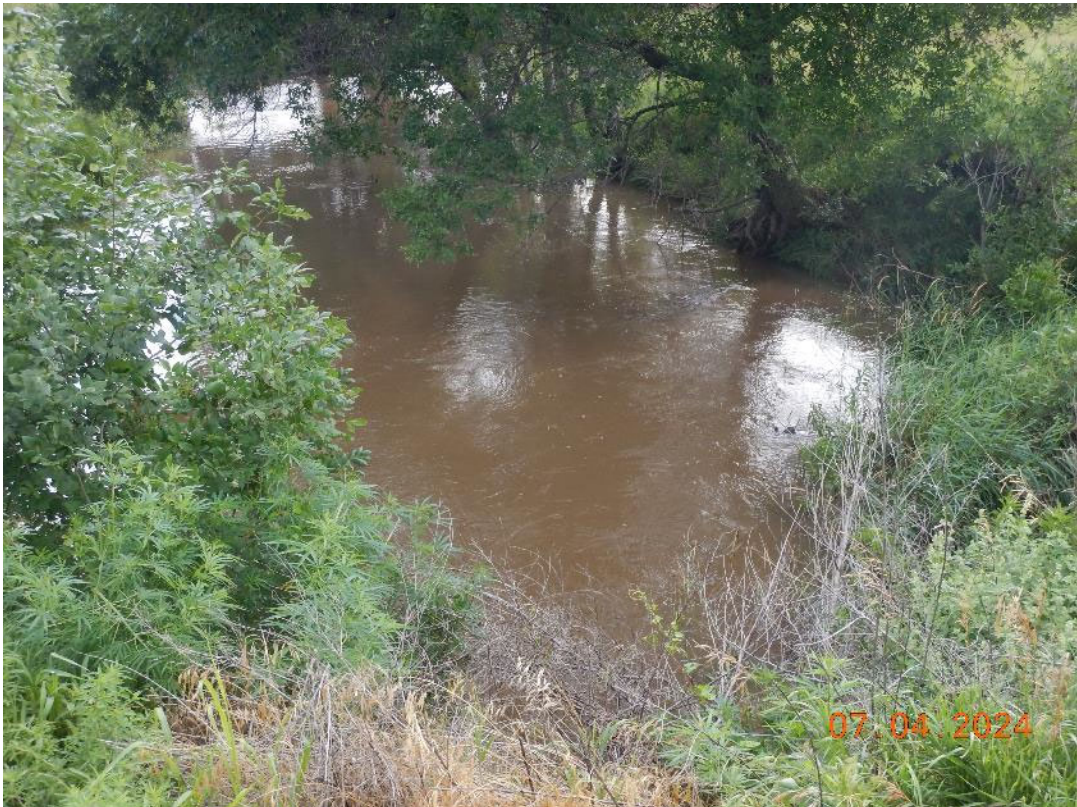
Photograph 14. Looking downstream from County Road 430 culvert.
