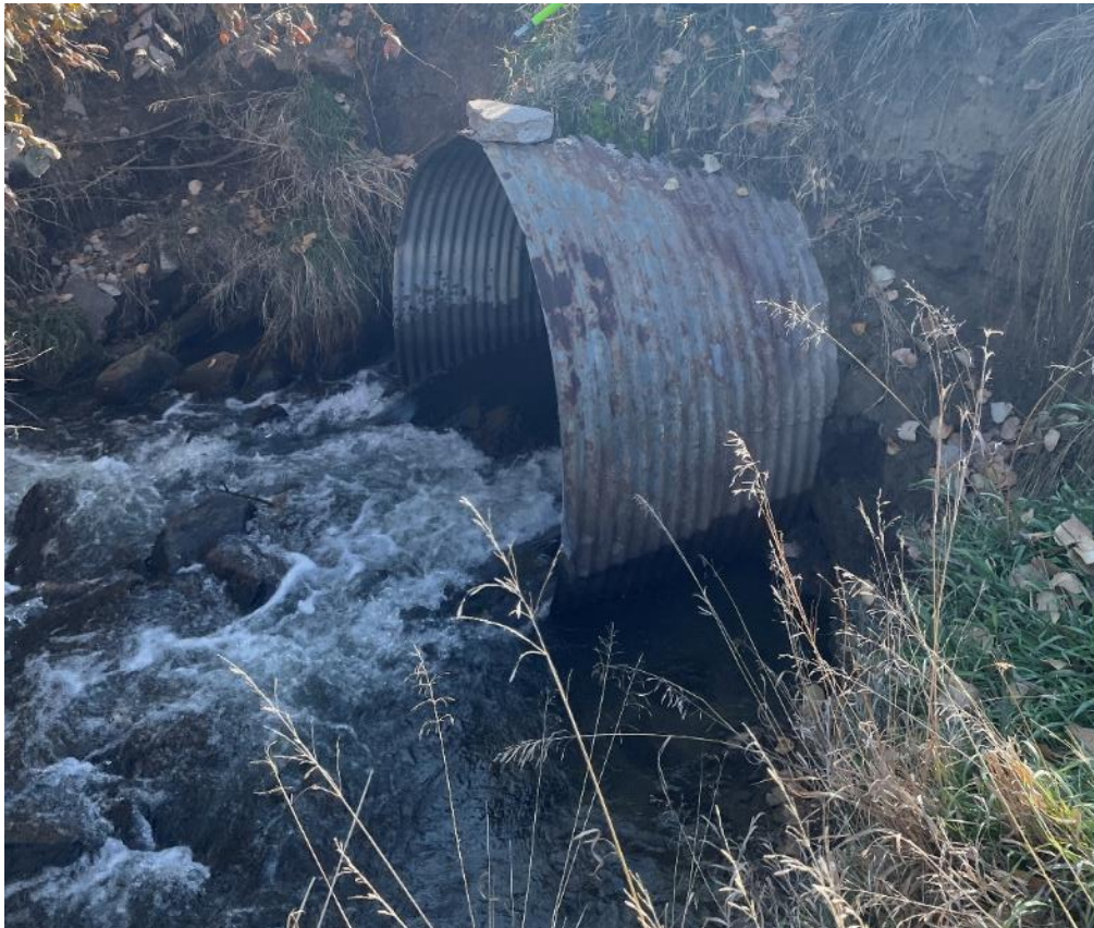
Figure 11: Typical culvert crossing on Plum Creek.
