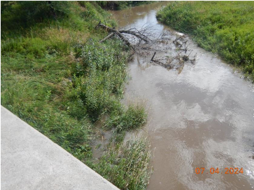
Photograph 18. Looking downstream from County Road 432 bridge.
