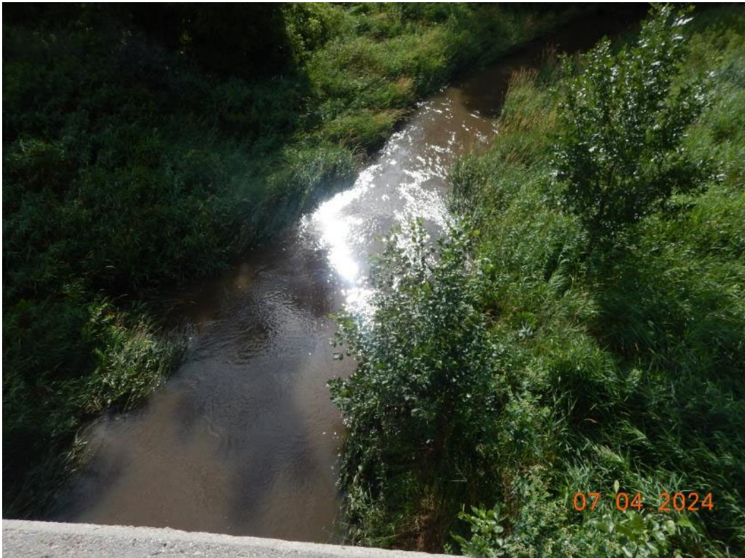
Photograph 4. Looking downstream from State Highway 283 bridge.
