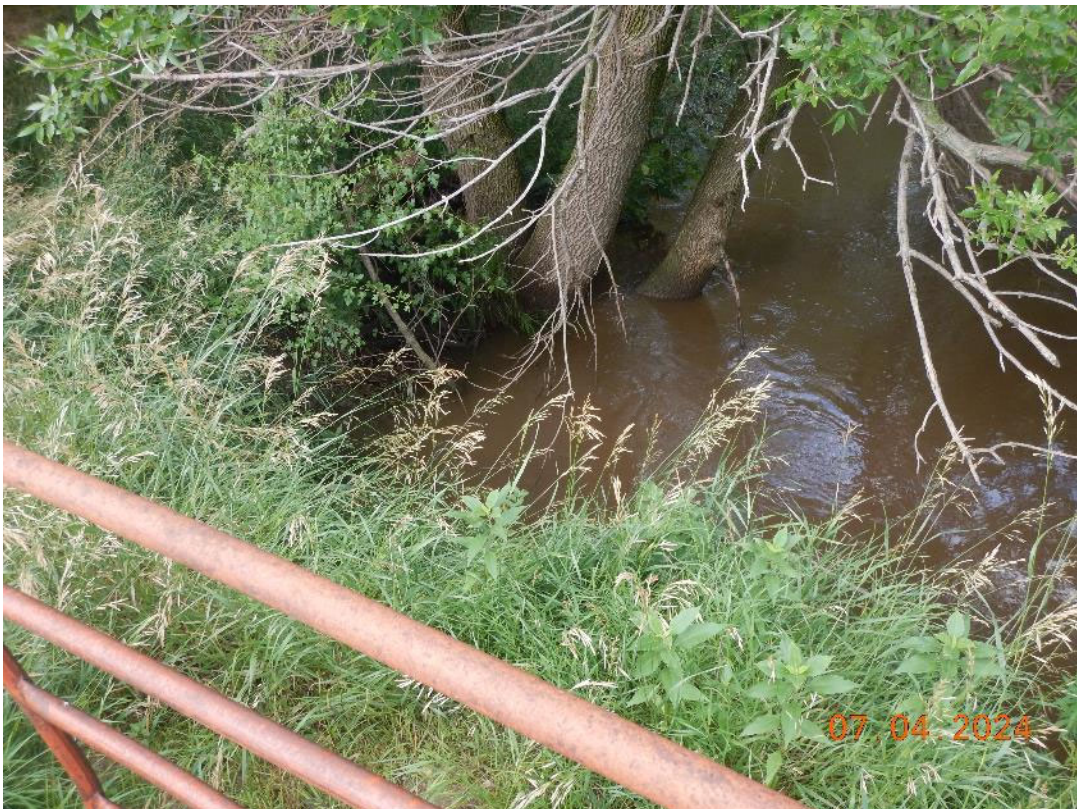
Photograph 10. Looking upstream from County Road 430 culvert.
