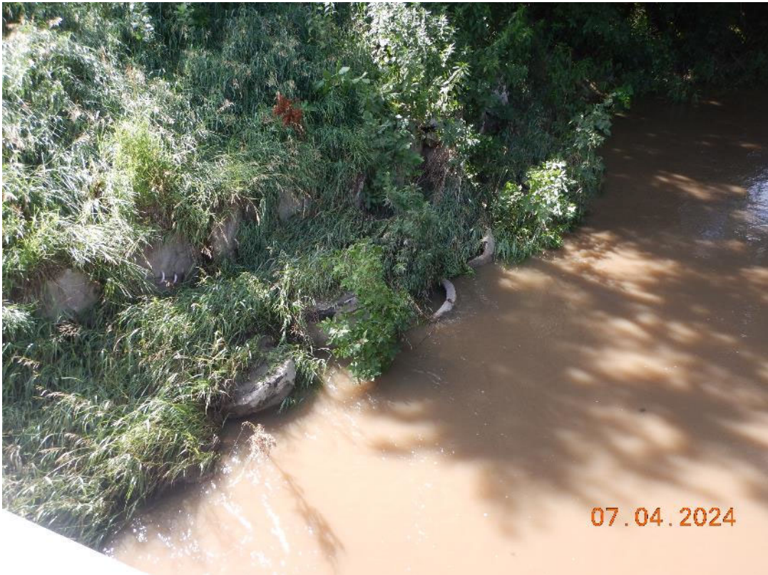
Photograph 26. Concrete blocks along streambank upstream of County Road 746 bridge.
