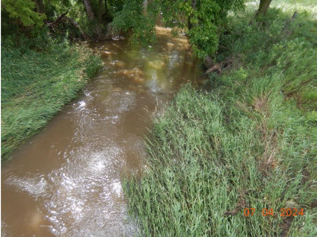
Photograph 9. Looking downstream from County Road 429 bridge.
