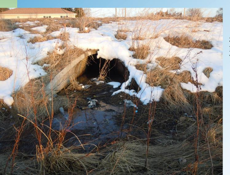
30" concrete pipe culvert with wingwall
