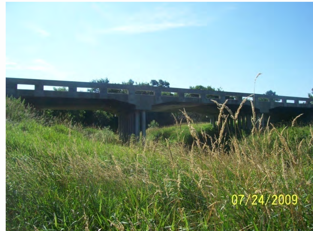
Photo 13. State Highway 283 bridge over Plum Creek, upstream face
