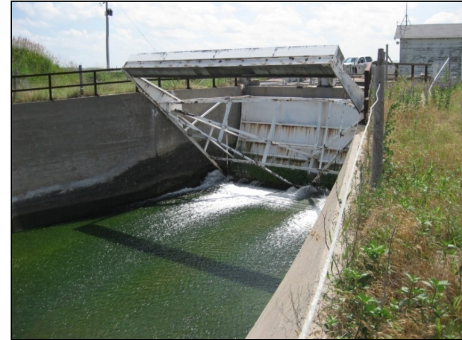
Photo 4.3-1 – J-2 Return Radial Gate, 30 feet wide by 13 feet, 6 inches tall
