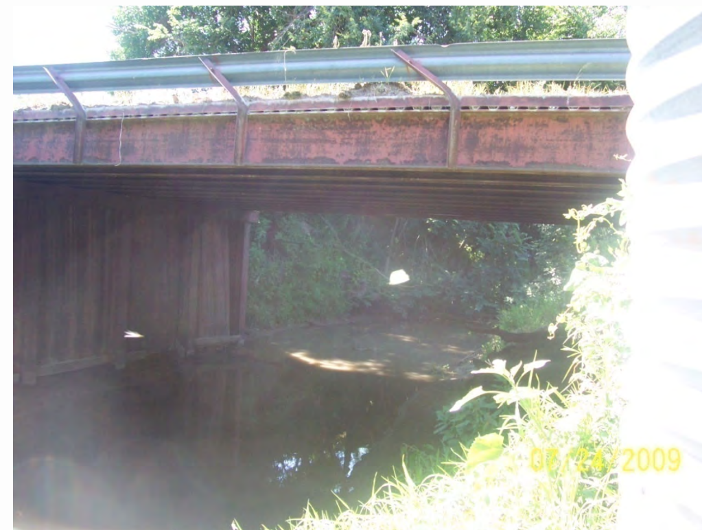
Photo 24. County Road 746 bridge over Plum Creek, downstream face
