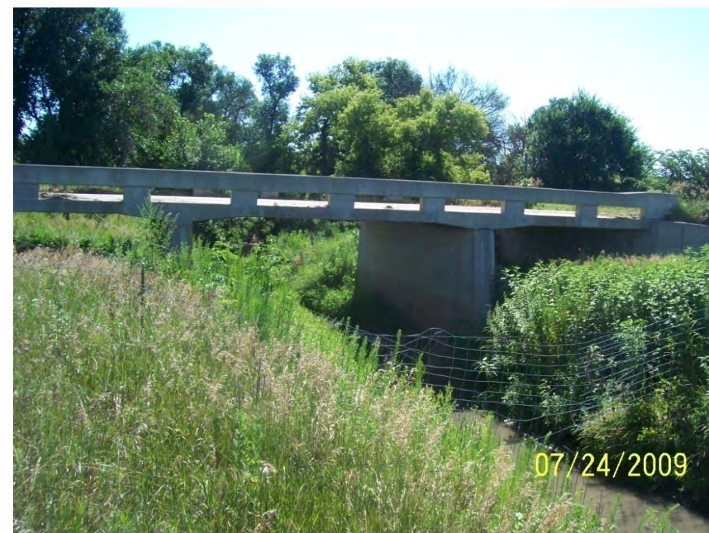
Photo 25. County Road 435 bridge over Plum Creek, upstream face
