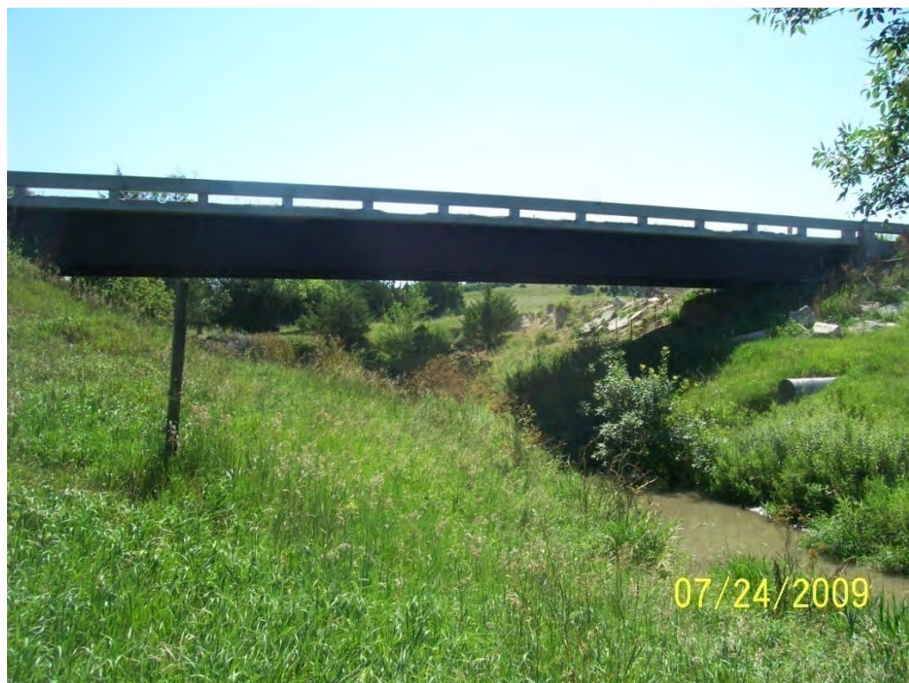
Photo 27. County Road 436 bridge over Plum Creek, upstream face
