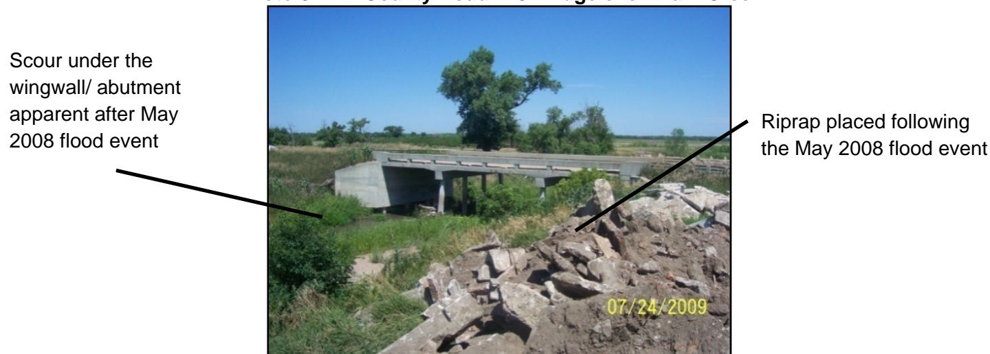
Photo 3.4-1 - County Road 749 Bridge over Plum Creek
