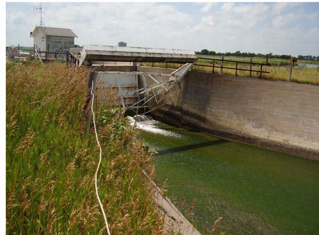
Photo 9. J2 wasting station
