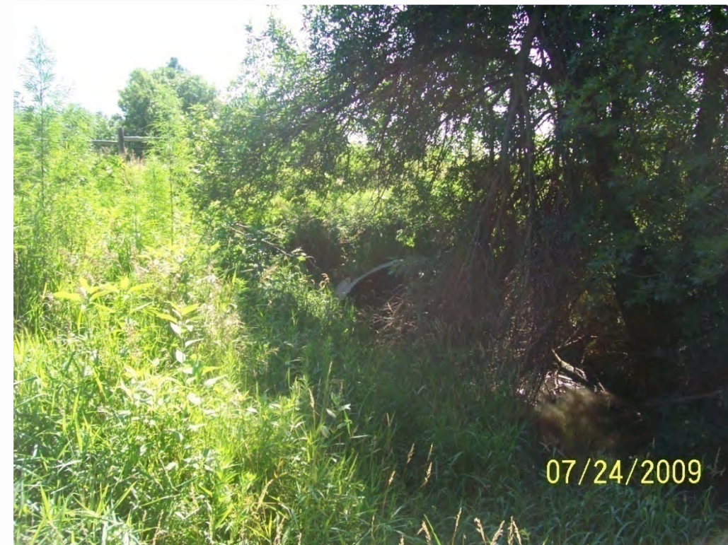
Photo 17. County Road 430 culvert in Plum Creek, upstream face
