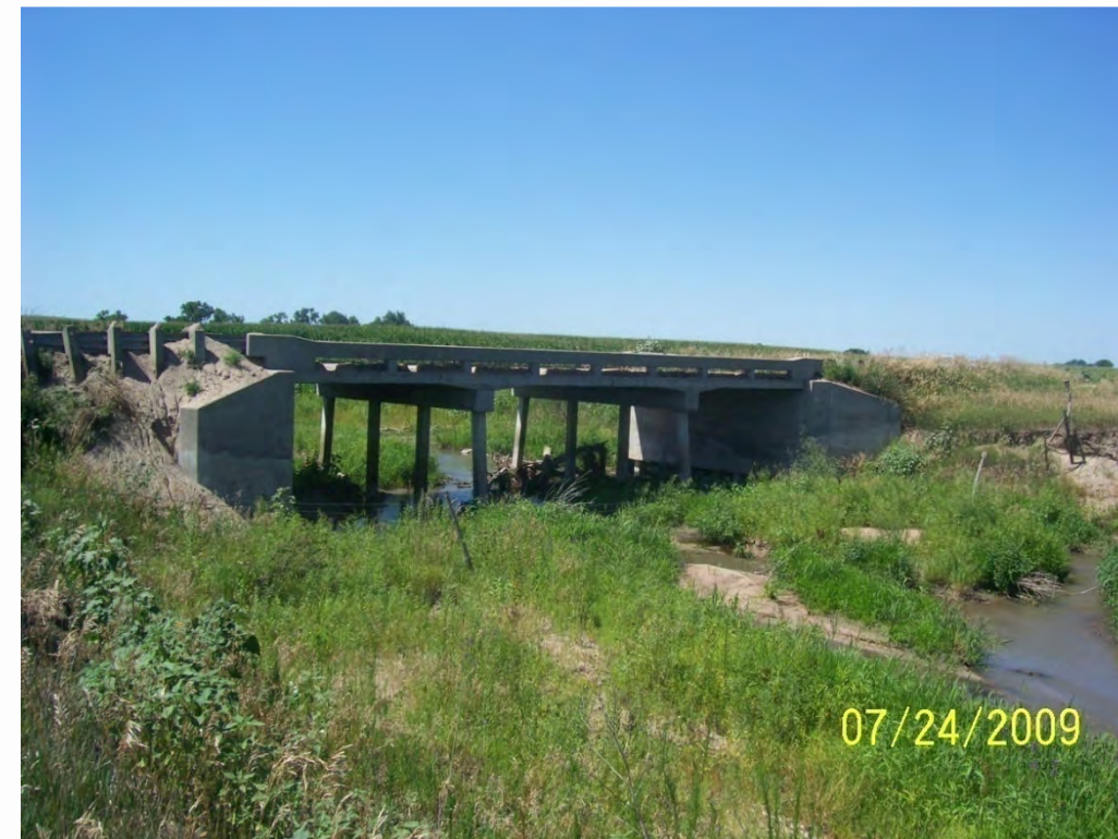
Photo 32. County Road 749 bridge over Plum Creek, downstream face
