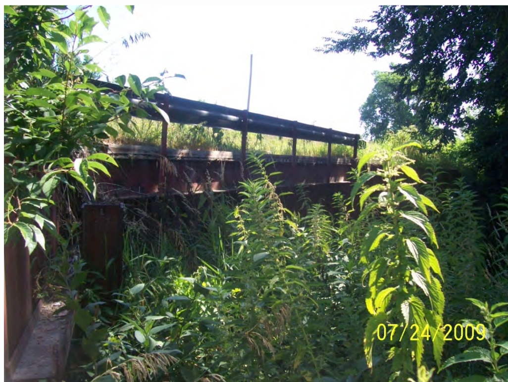
Photo 23. County Road 746 bridge over Plum Creek, upstream face
