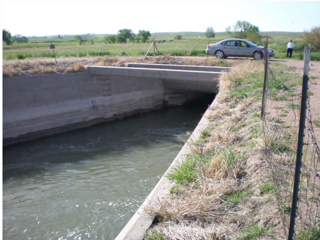
Photo 6. Phelps Canal siphon at Plum Creek
