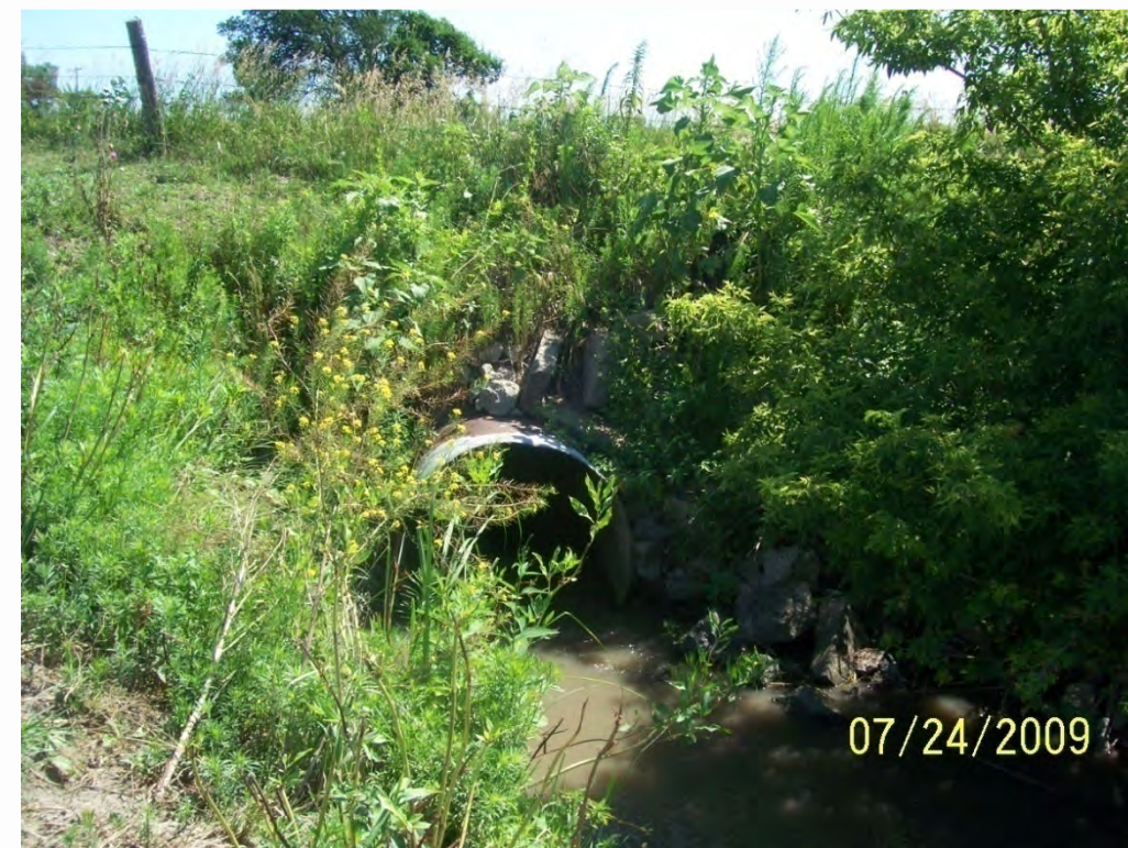
Photo 29. County Road 437 culvert in Plum Creek, upstream face
