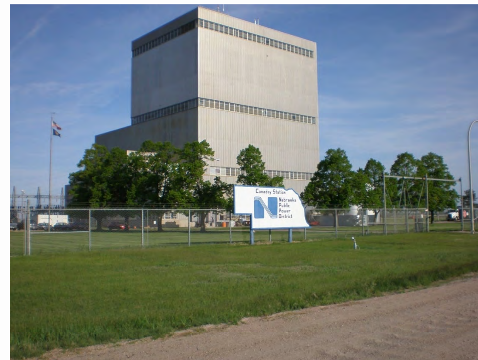
Photo 33, NPPD Canaday Station steam power plant
