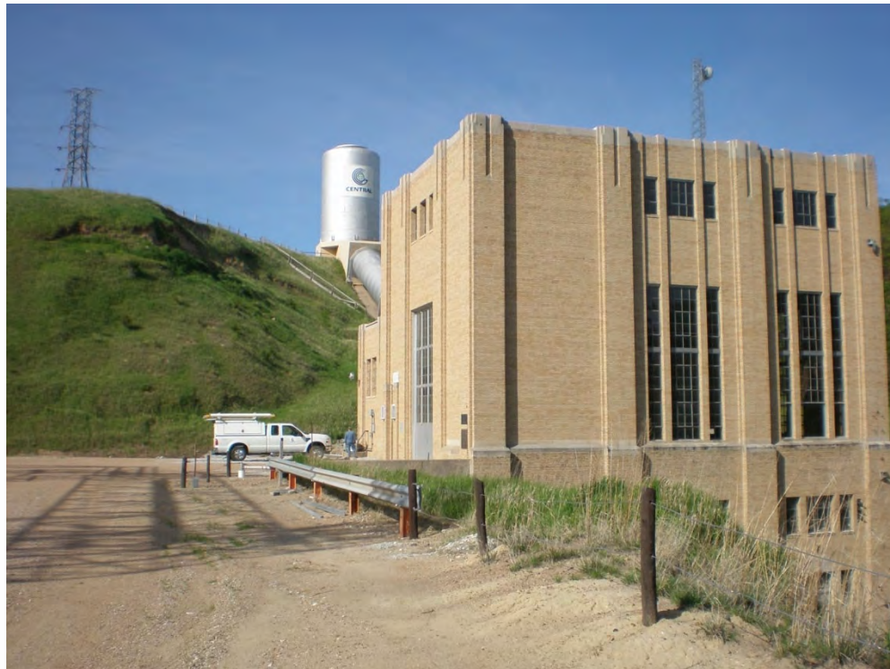
Photo 39, CNPPID J-2 Hydropower station
