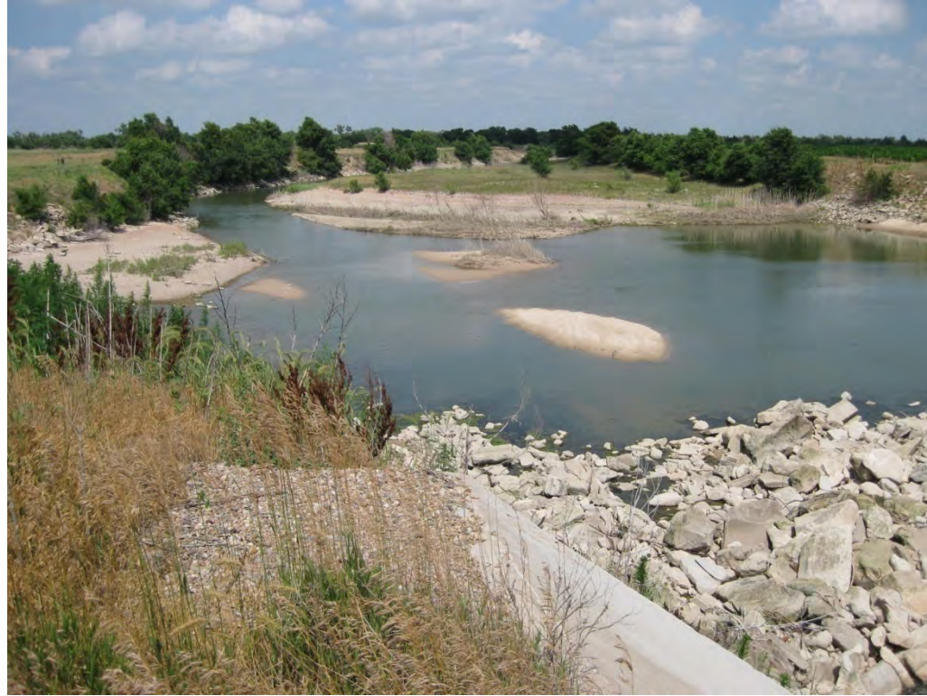
Photo 10. J2 below the J-2 Wasting Station
