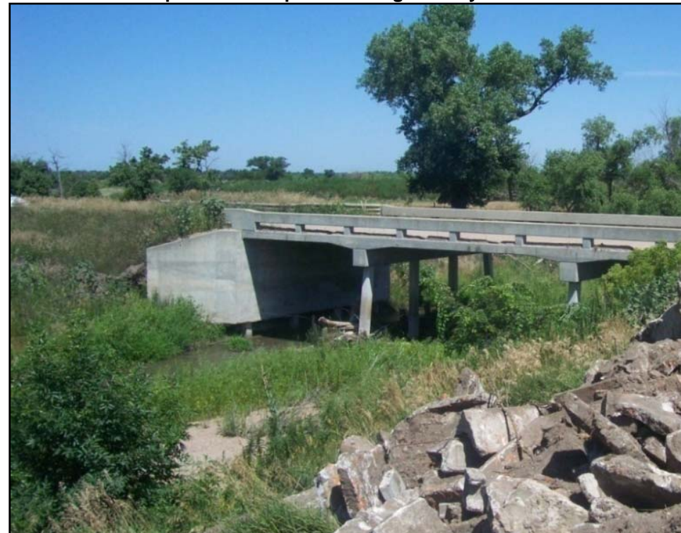
Photo 4.3-2 – County Road 749 Bridge over Plum Creek. West abutment piers were exposed during the May 2008 flood event.
