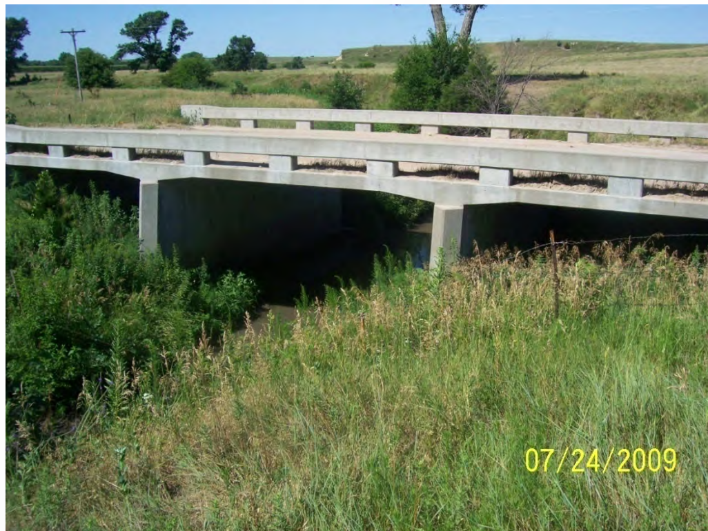
Photo 26. County Road 435 bridge over Plum Creek, downstream face
