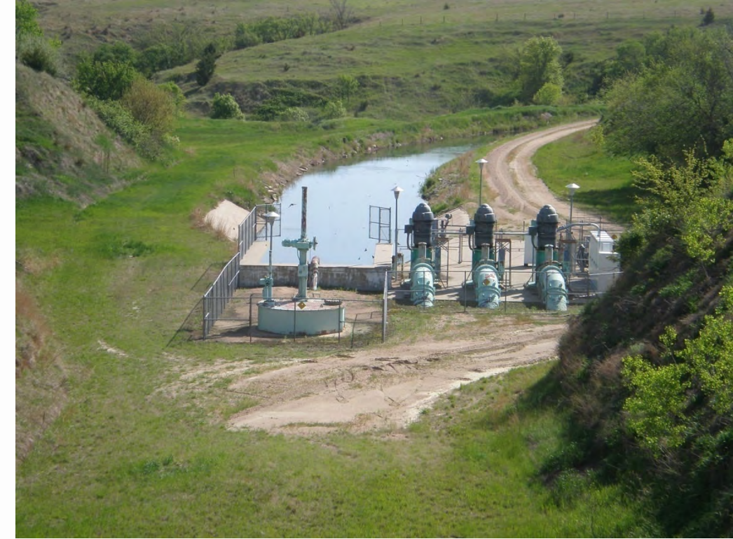
Photo 3. Elwood Reservoir pump station
