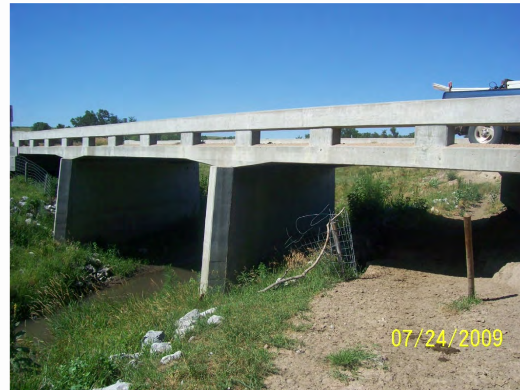
Photo 20. County Road 432 bridge over Plum Creek, downstream face
