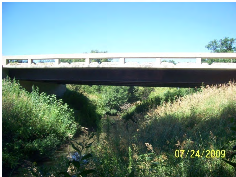
Photo 22. County Road 433 bridge over Plum Creek, downstream face
