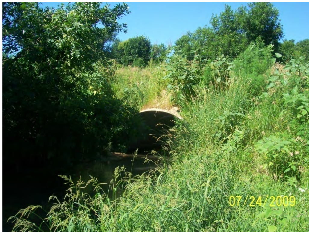
Photo 18. County Road 430 culvert in Plum Creek, downstream face
