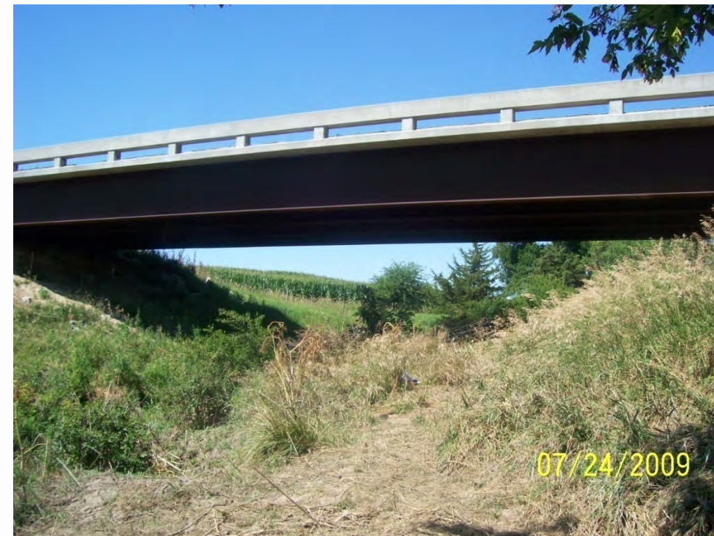
Photo 28. County Road 436 bridge over Plum Creek, downstream face
