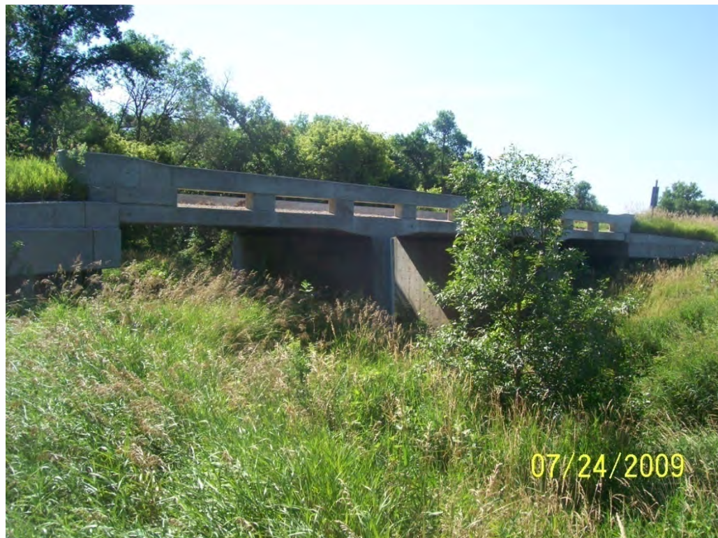
Photo 15. County Road 429 bridge over Plum Creek, upstream face
