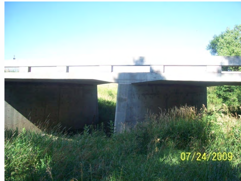
Photo 16. County Road 429 bridge over Plum Creek, downstream face
