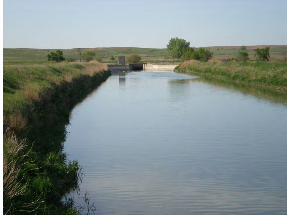
Photo 38, Approach to the Phelps Canal siphon under Plum Creek
