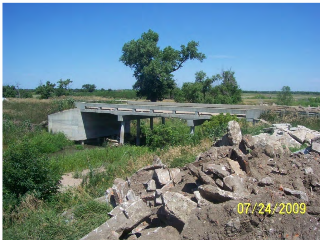
Photo 31. County Road 749 bridge over Plum Creek, upstream face
