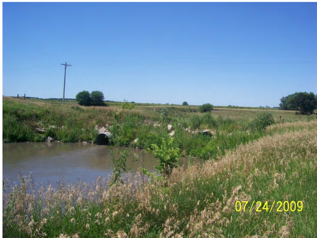
Photo 30. County Road 437 culvert in Plum Creek, downstream face
