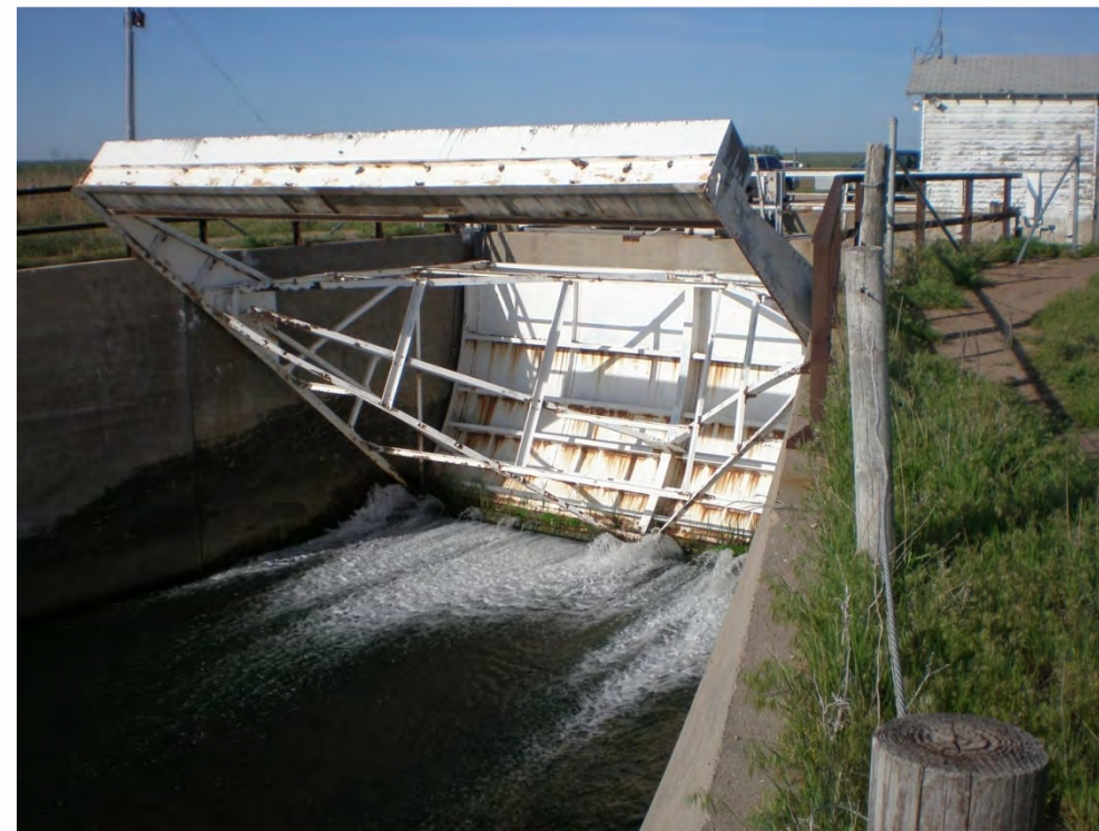
Photo 36, J-2 Return wasting station radial gate discharge to the south channel of the Platte River
