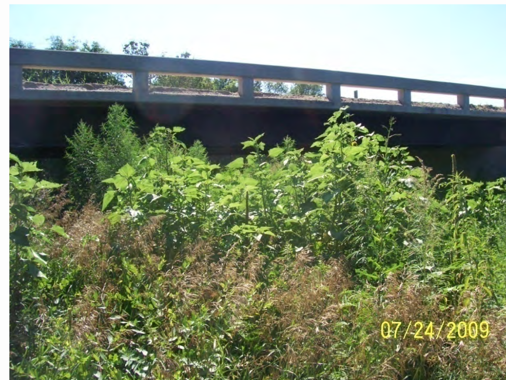
Photo 21. County Road 433 bridge over Plum Creek, upstream face
