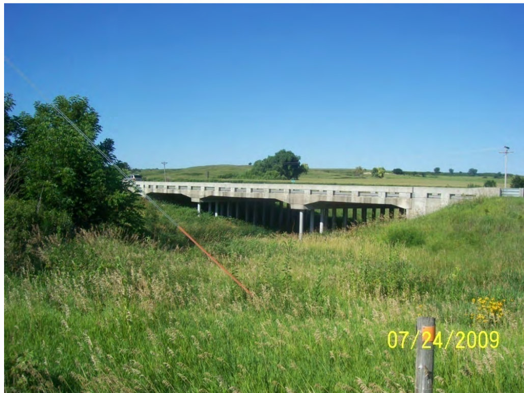
Photo 14. State Highway 283 bridge over Plum Creek, downstream face
