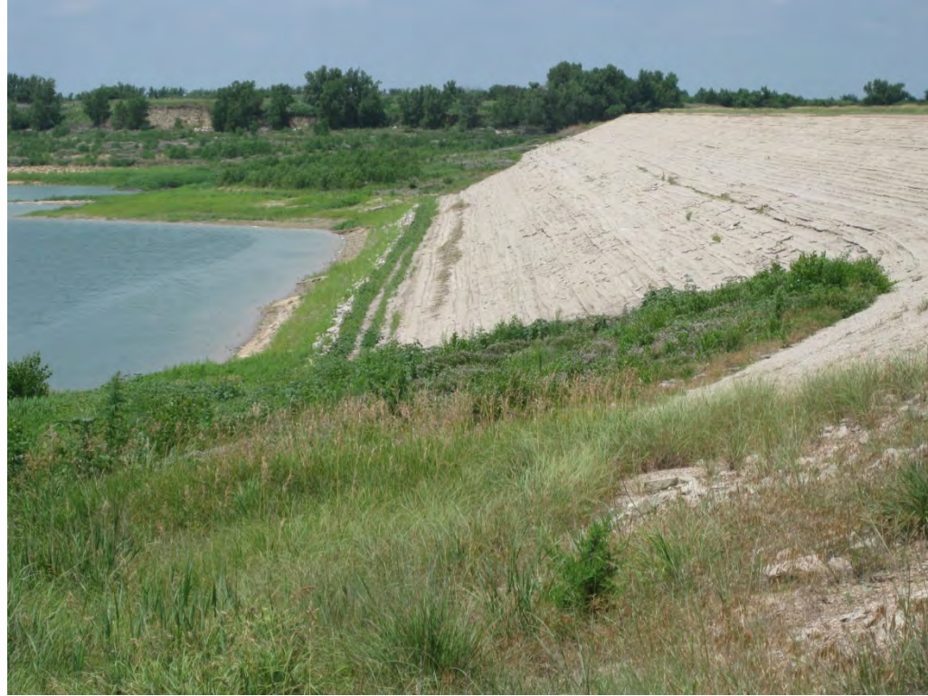
Photo 1. Elwood Reservoir dam
