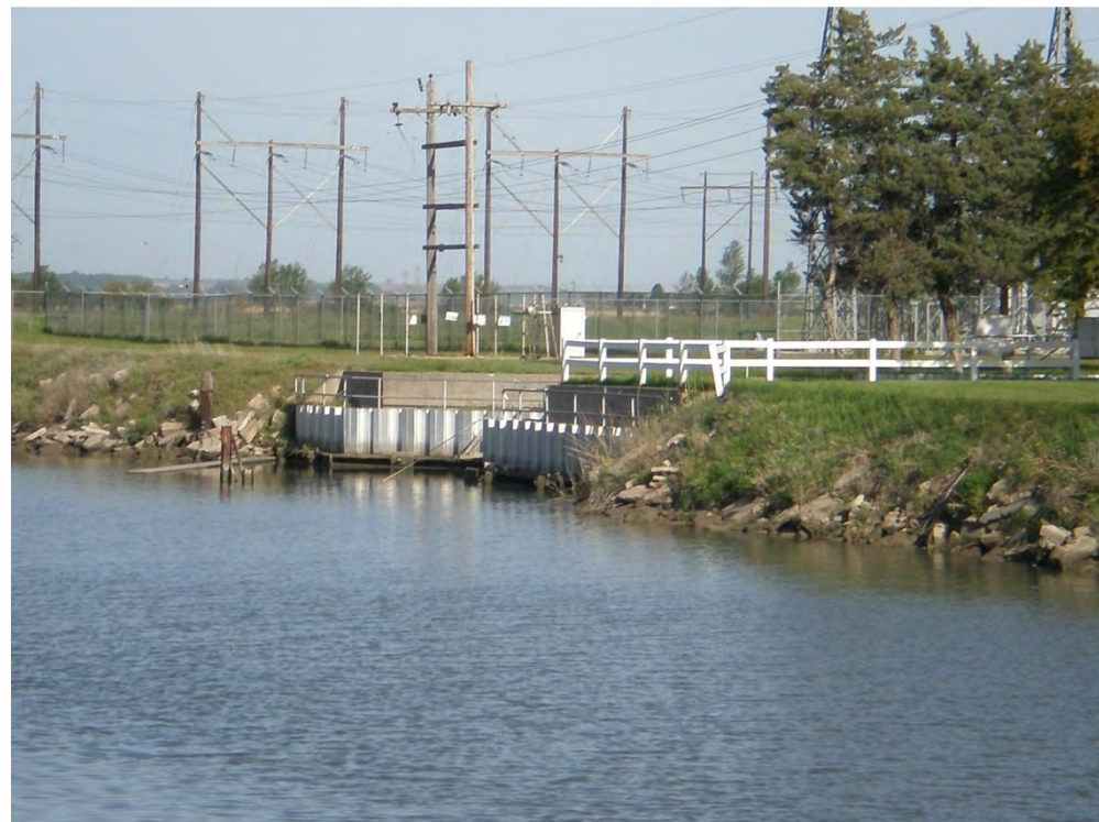
Photo 34, NPPD Canaday Station steam power plant cooling water intake on J-2 Return Canal
