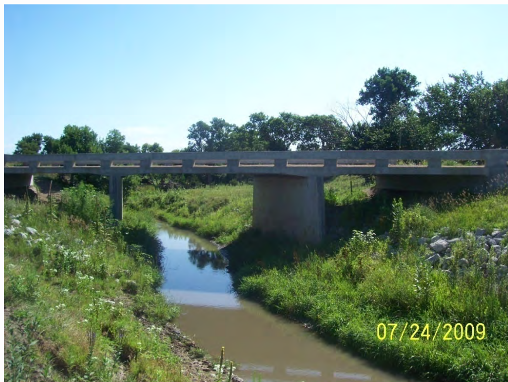
Photo 19. County Road 432 bridge over Plum Creek, upstream face
