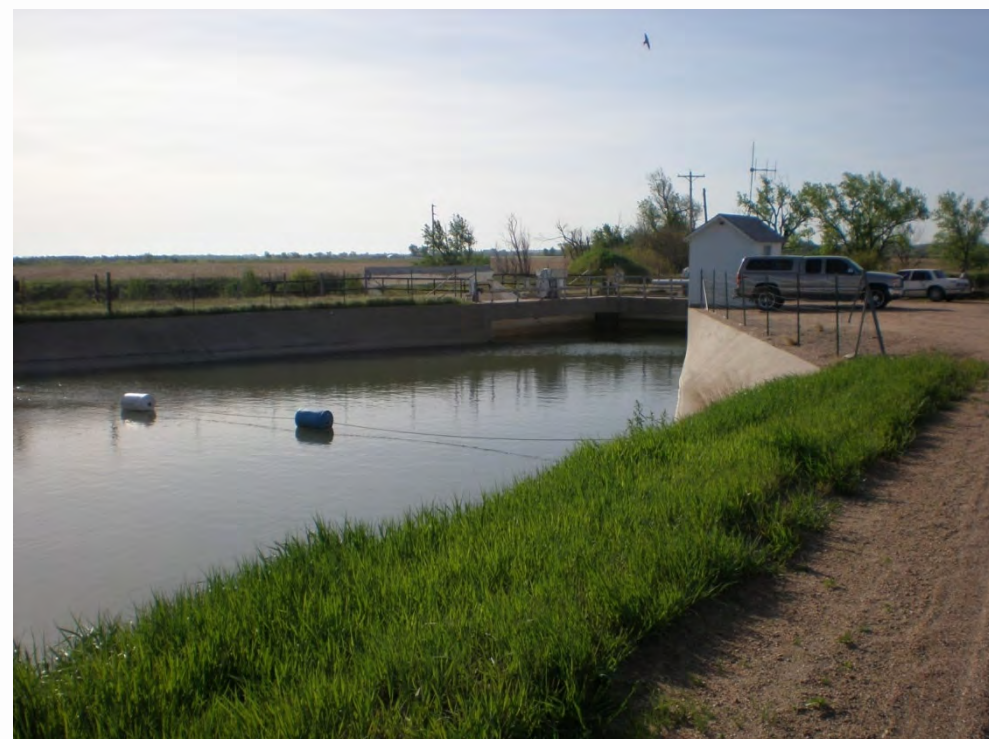
Photo 35, Approach to J-2 Return wasting station
