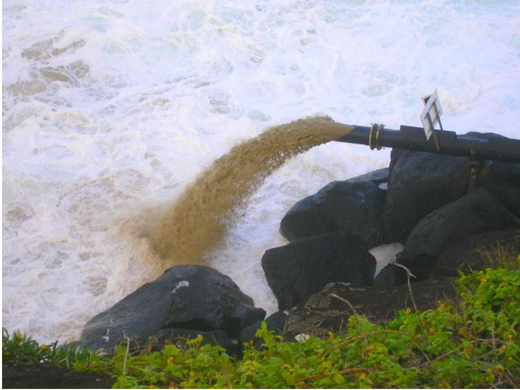
Figure 7-9 Discharging Sediment Directly to River
