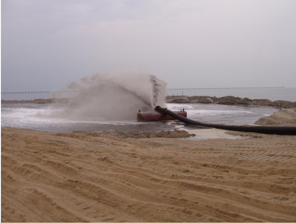
Figure 7-5 Slurry Pipeline Delivering Sand
