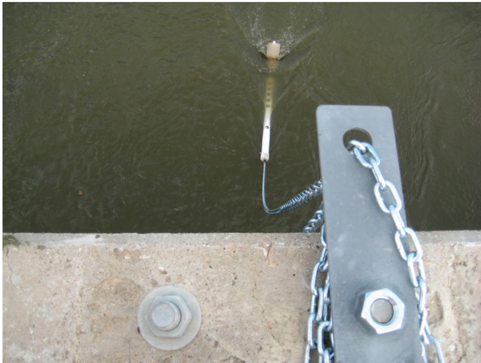
9. Log chain attachment to bridge deck near Kearney, NE.
