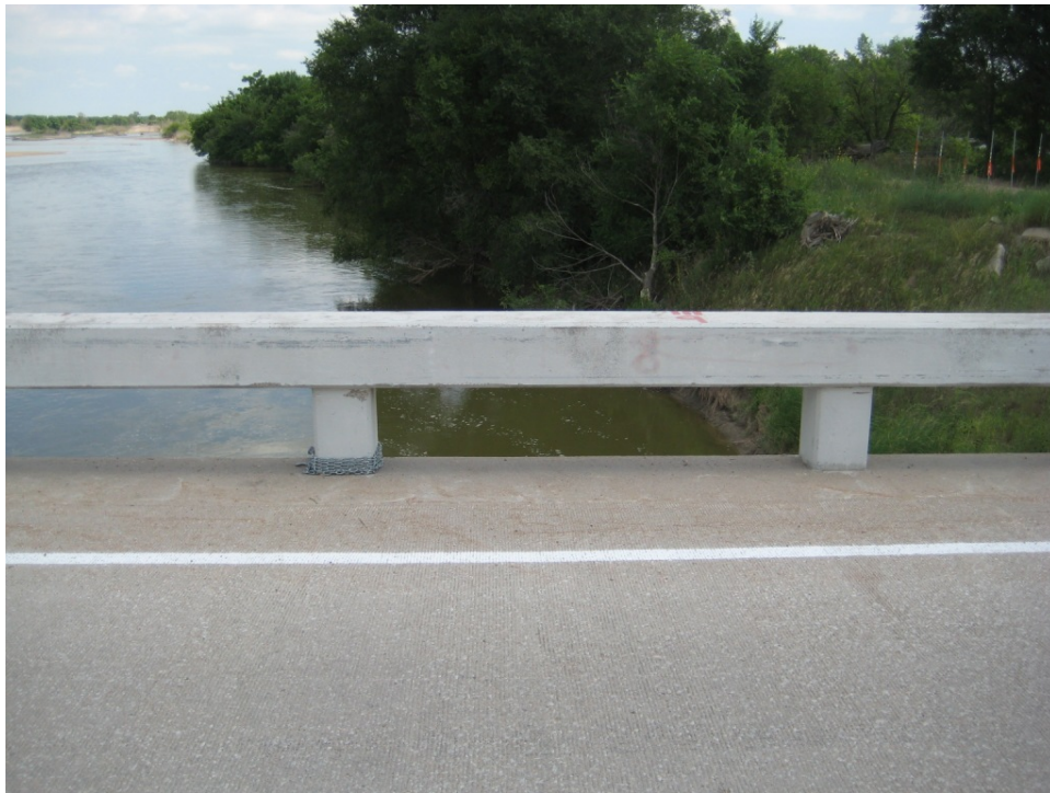
7. Log chain attachment to bridge deck near Duncan, NE.
