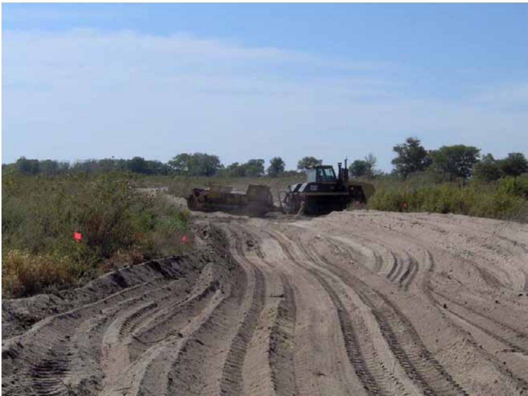
Figure 1.3. Construction of a side channel on the left bank of habitat site 6.
