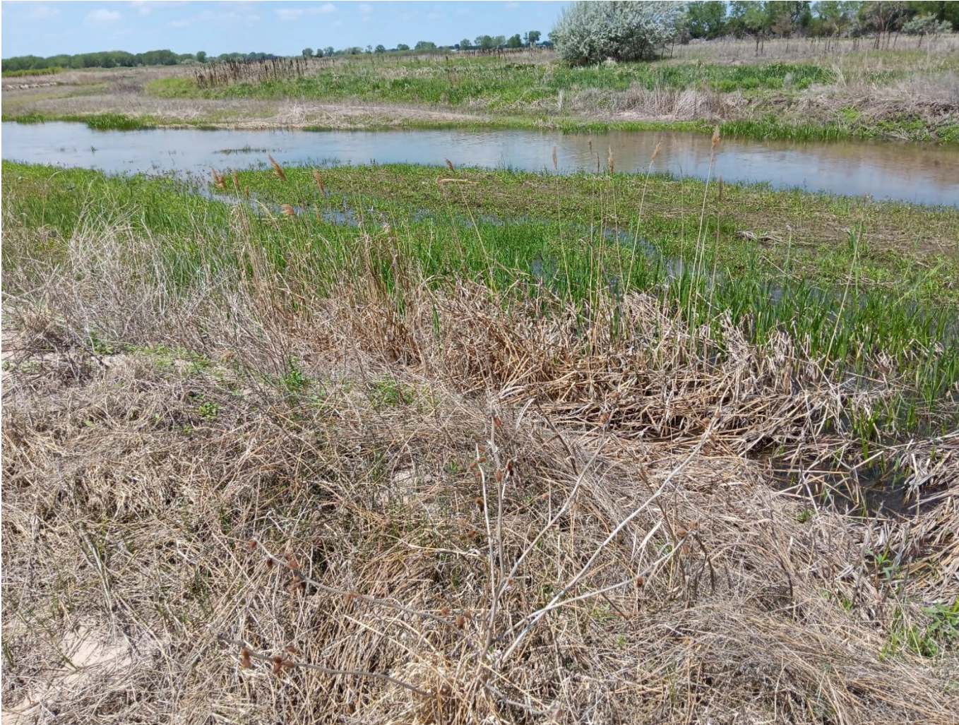
Figure 9. Photo of the bankline patch (in foreground) corresponding to the patch depicted in Figure 8. This photo was taken on the southeast corner of the patch and facing to the northwest.
